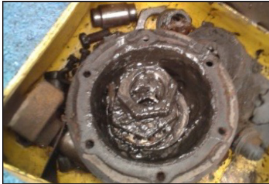
Marine port equipment stopped due to failed bearings and insufficient greasing.
